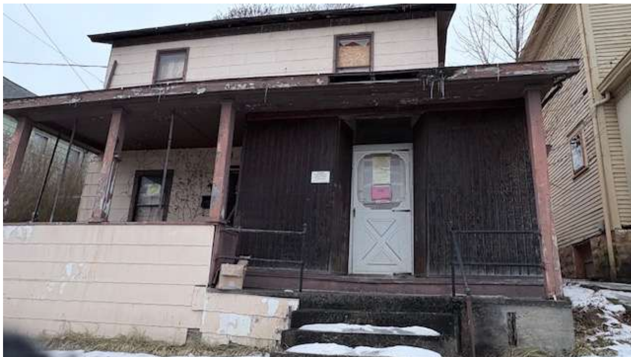
Demolition – 1003 East Second Street, Oil City PA
